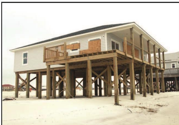
Figure 7.14: Pile Foundations
